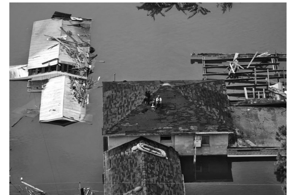
Homes are flooded to the roof from Hurricane Katrina.
